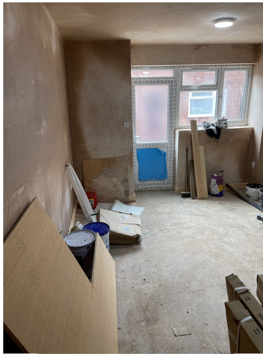
Internal View of Ground Floor
