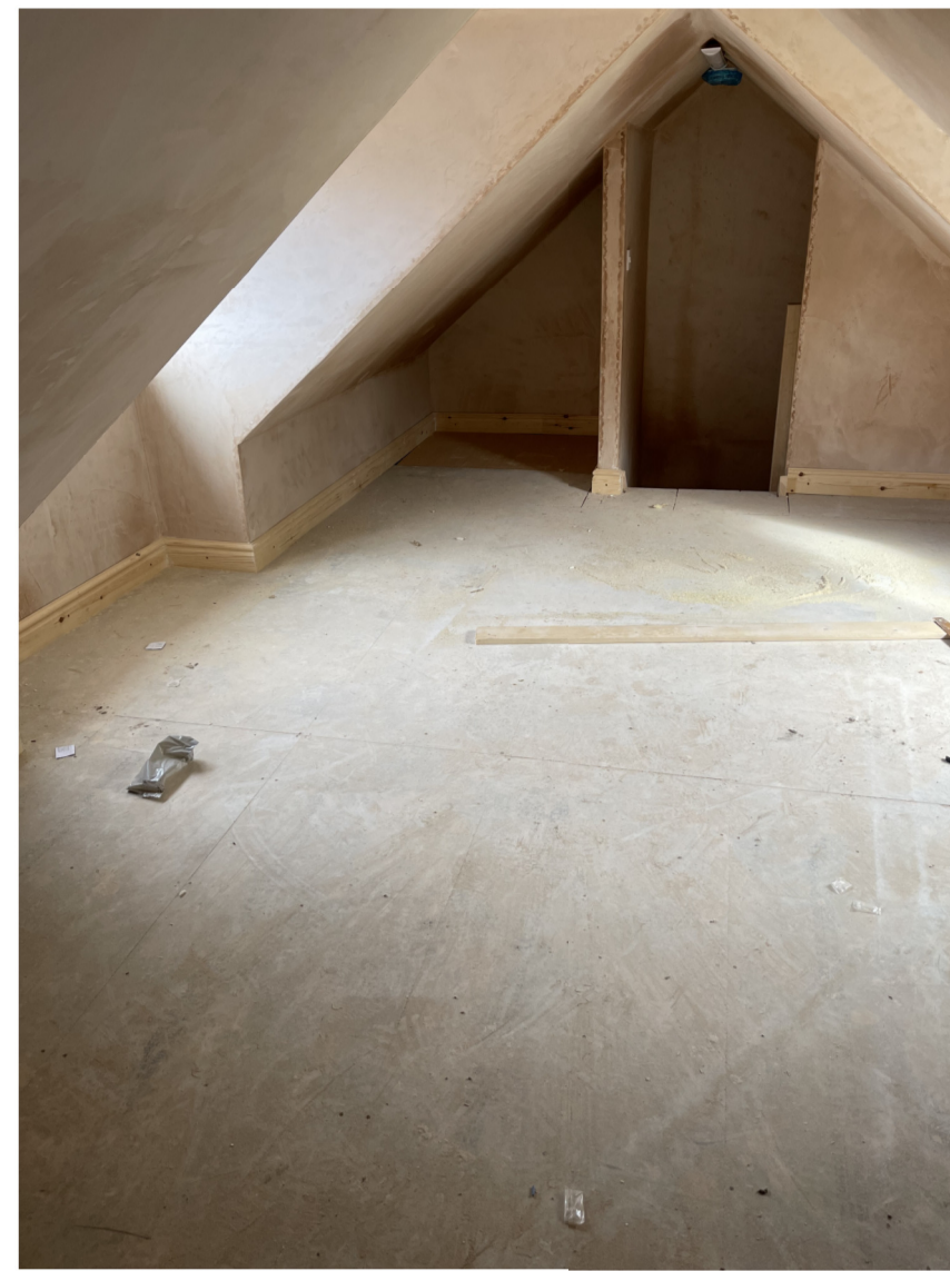
Internal View of First Floor
